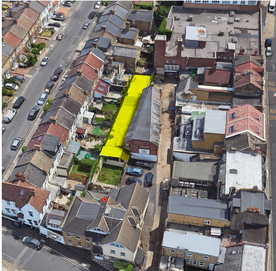
Figure 2 – Aerial view (building as existing highlighted yellow)
