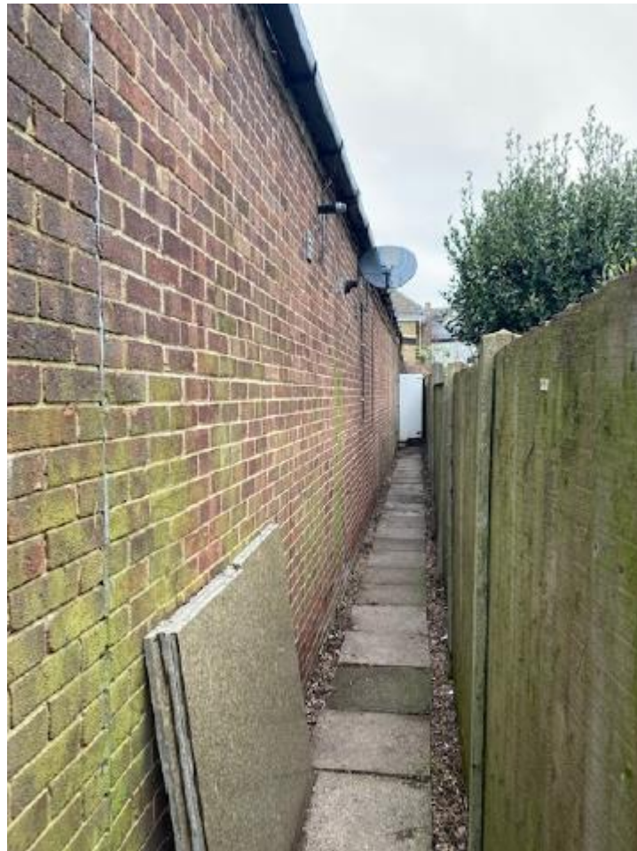
Figure 4 Rear alleyway as existing
